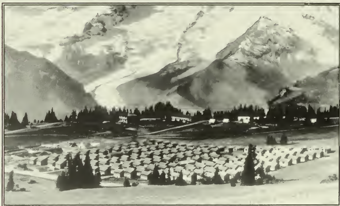
Sunrise housekeeping cabins built in 1930 and removed in 1943-44. Damage to the sensitive subalpine meadow is still visible. (Tahoma Woods Collection)
